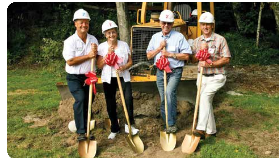
Bob Ecklund, YMCA President and CEO, with Deanna Dally, Ray Dally, and Jim Carmichael at the YMCA Camp Seymour Dining Hall Groundbreaking.
