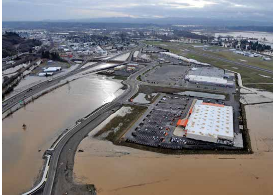
Flood waters turn Chehalis Wal-Mart and Home Depot parking lots into islands. I-5 is in the upper left.
