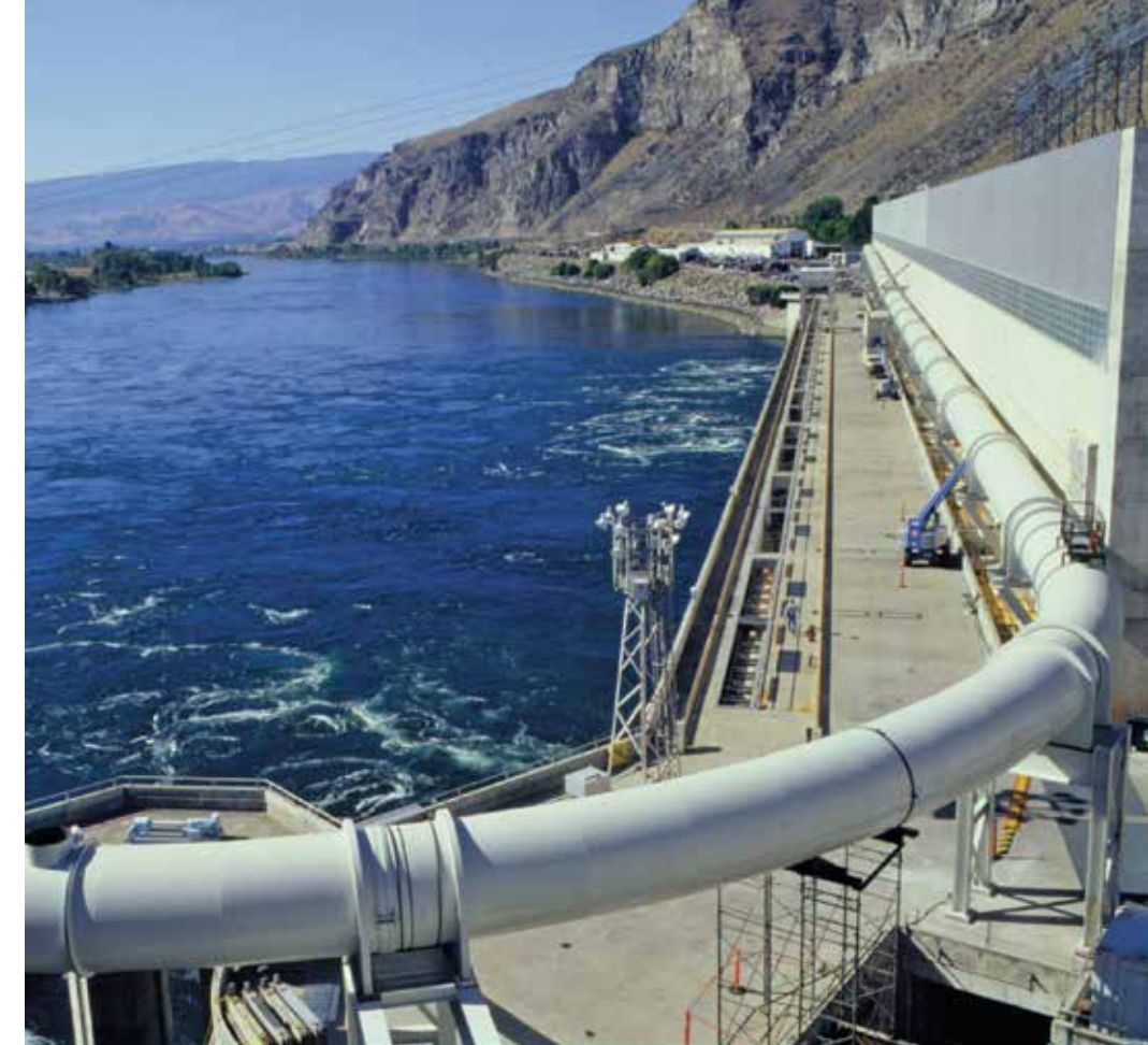
In 2003, Chelan PUD installed a first-of-its-kind juvenile fish bypass system to help young salmon and steelhead around the dam on their way to the ocean.
