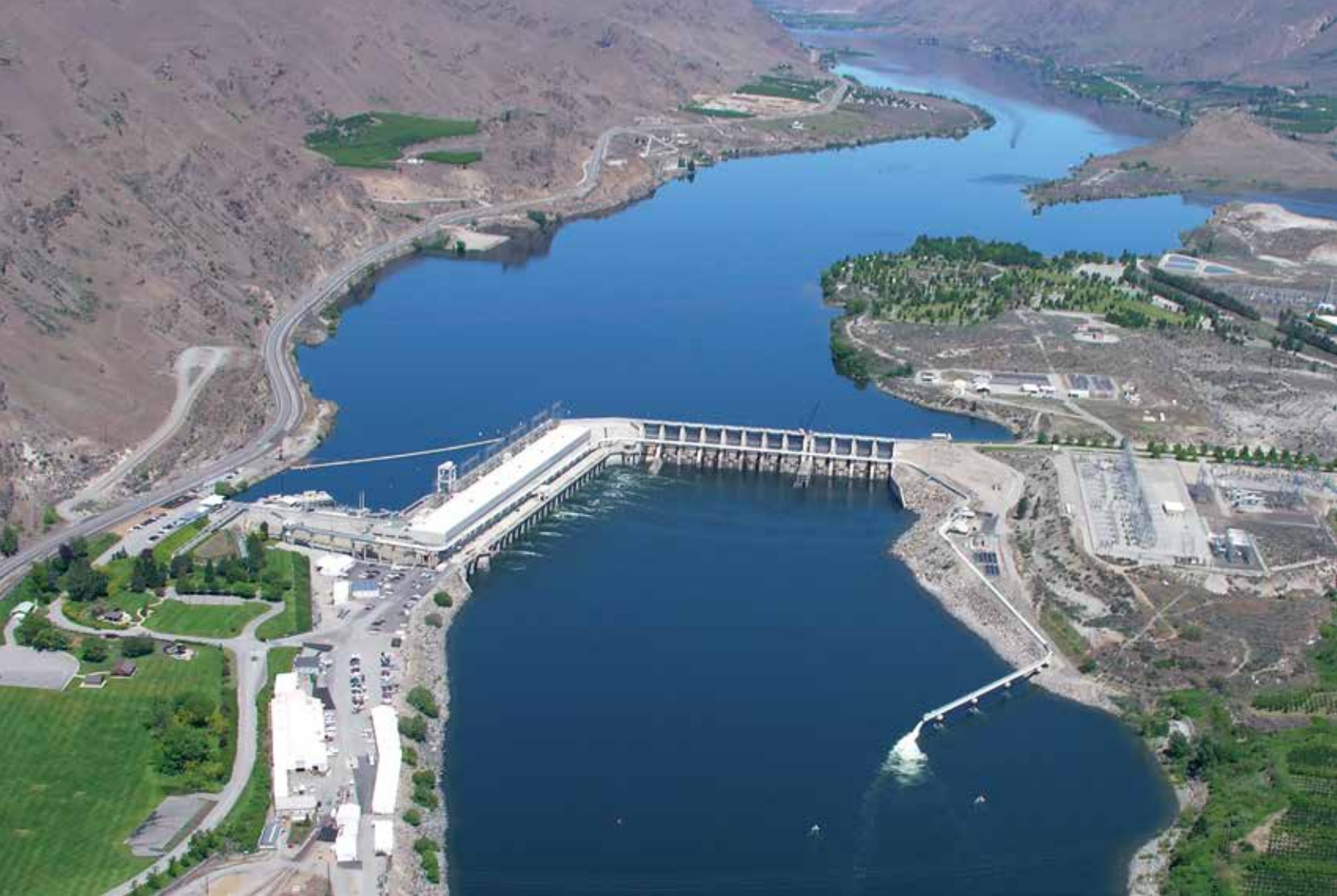
Rocky Reach Dam straddles the Columbia River seven miles north of Wenatchee. More than 7 million people throughout the Northwest benefit from clean, renewable energy produced by the Rocky Reach Hydroelectric Project.
